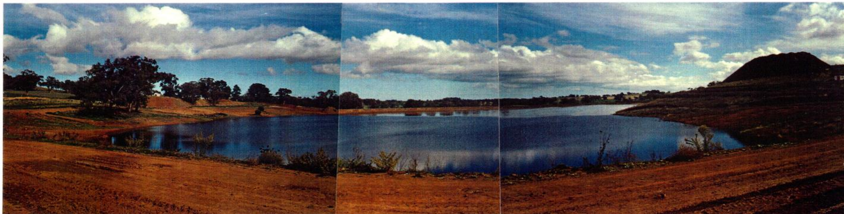
Plate 4: View of the tailings disposal facility looking southwest from the saddle dam. Waste rock stockpiled for later spreading during rehabilitation, is evident to the north and south (May 1989). (Ref: 127K/5,6,7)
