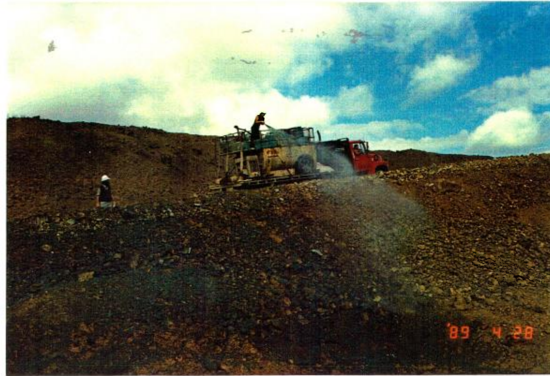
Plate 8: Hydromulching (native shrub seed and wood pulp) trial on exposed waste rock batter (April 1989). (Ref: 127J/18)
